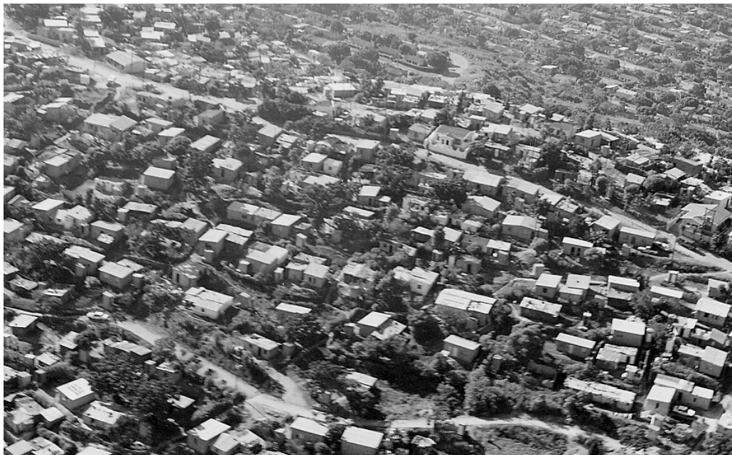
Figure 7: High density areas typical of many distribution areas
