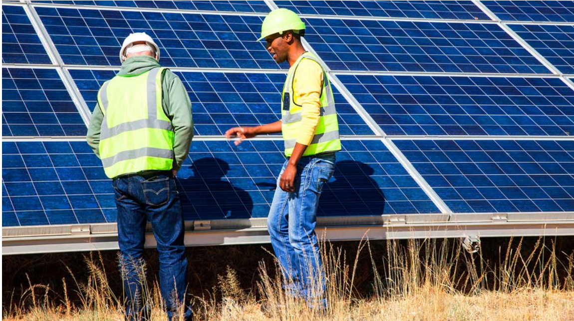
Droogfontein solar power PV plant near Kimberley
