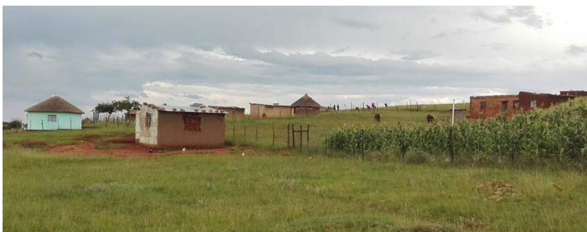
Figure 2: Solar Home systems in Matatiele, Eastern Cape
