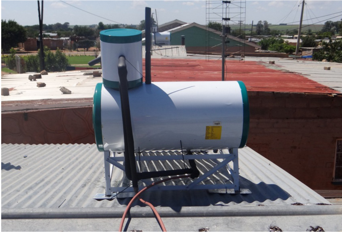
Figure 9: Low pressure SWH system
