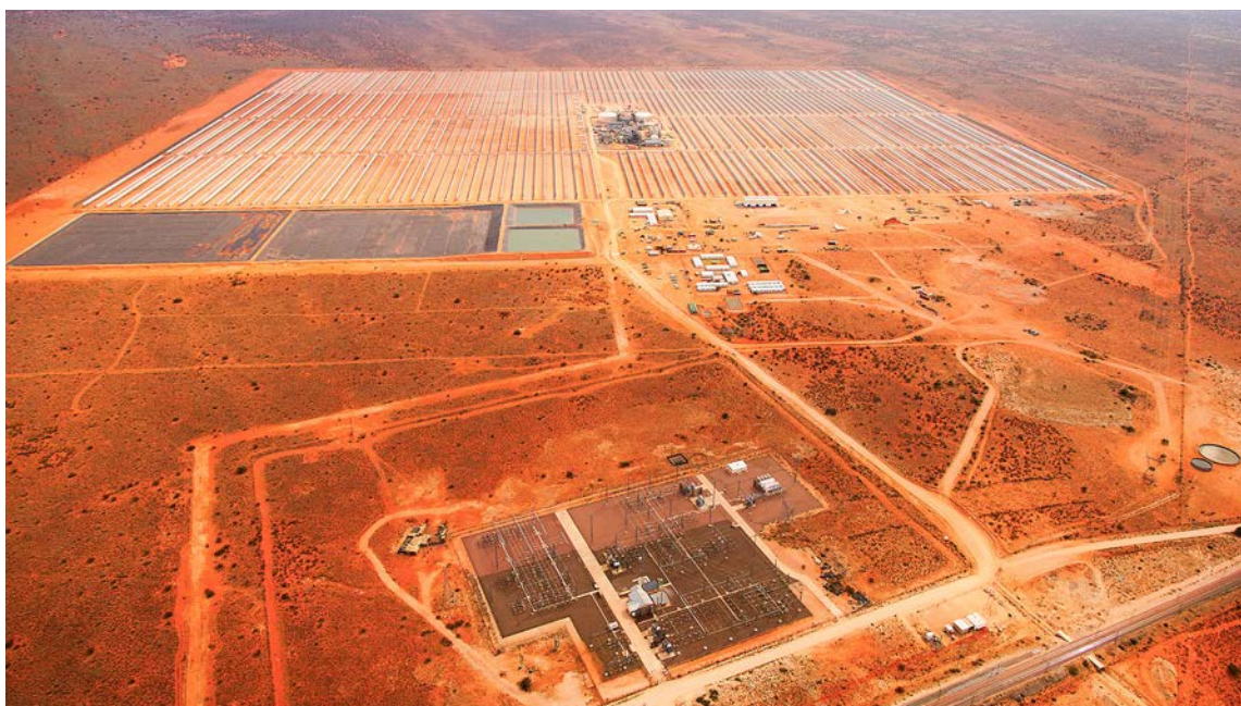
Bokpoort concentrated solar power plant near Groblershoop
