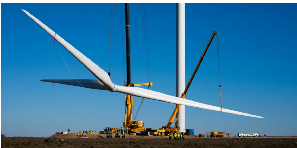
Wind turbine being assembled
