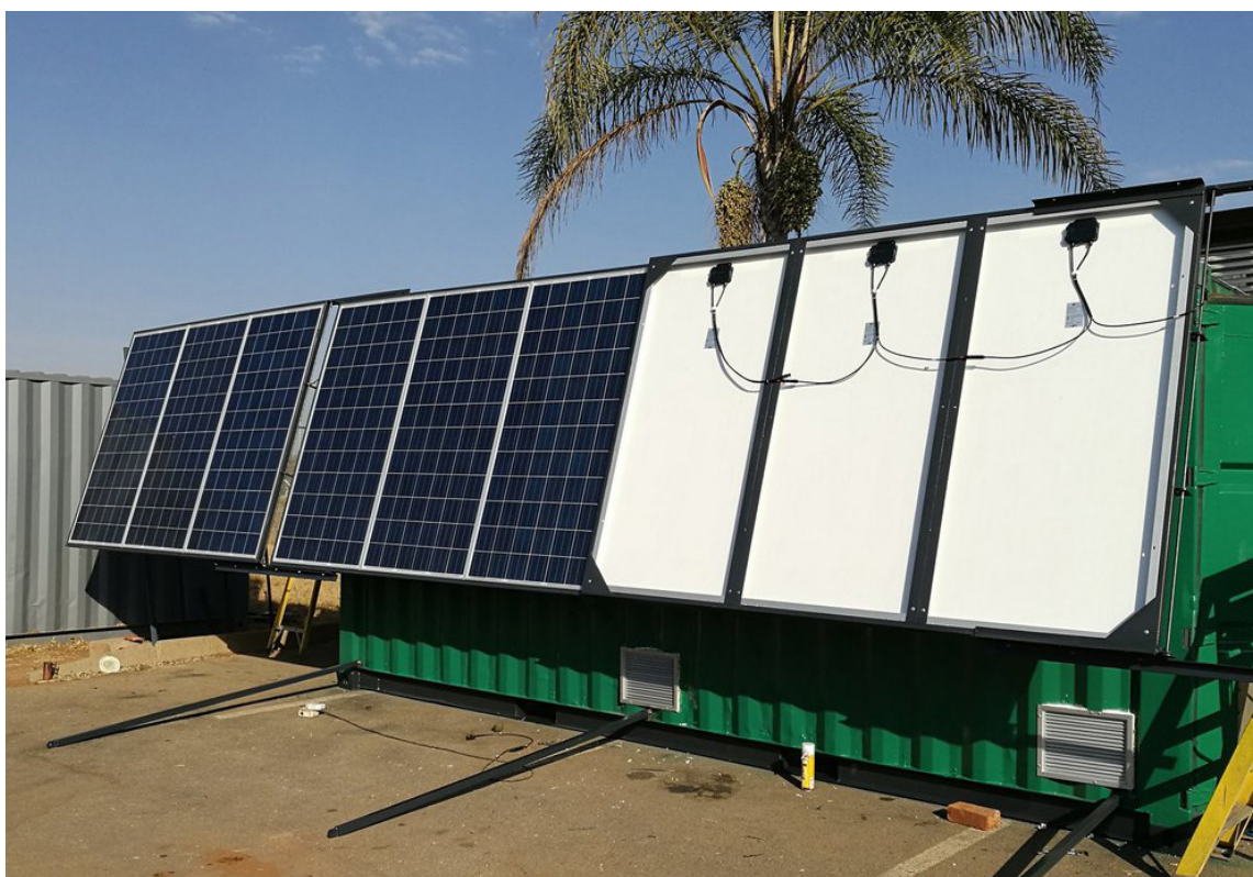
Figure 11: SolarTurtle container with partially unfolded PV panels (photo sourced from SolarTurtle Twitter feed)
