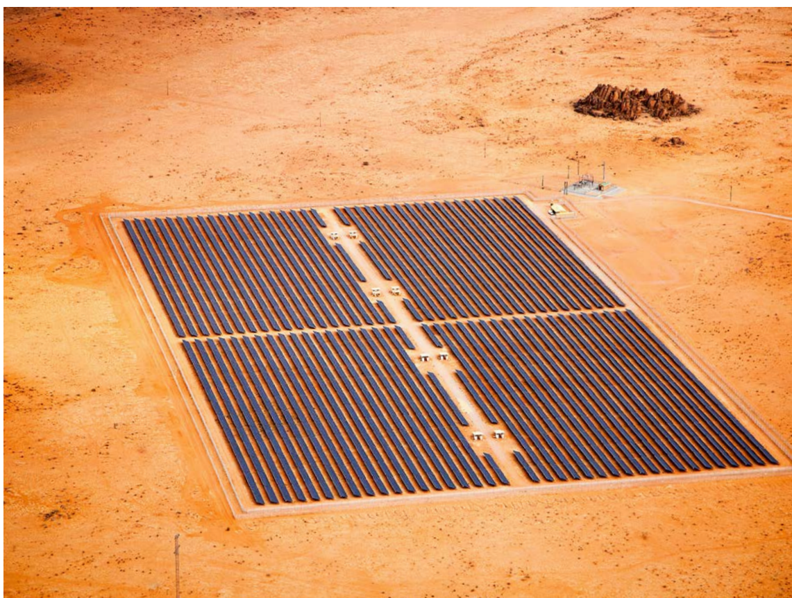
BioTherm Energy Konkoonsies solar PV plant near Pofadder
