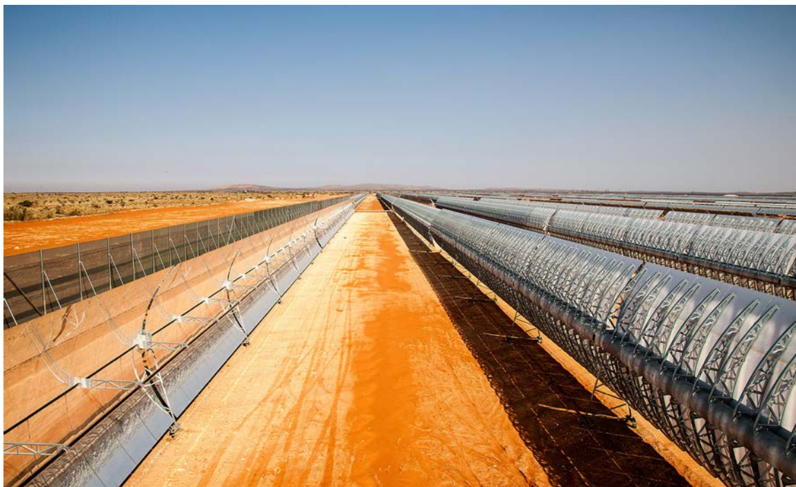
Bokpoort concentrated solar power plant near Groblershoop
