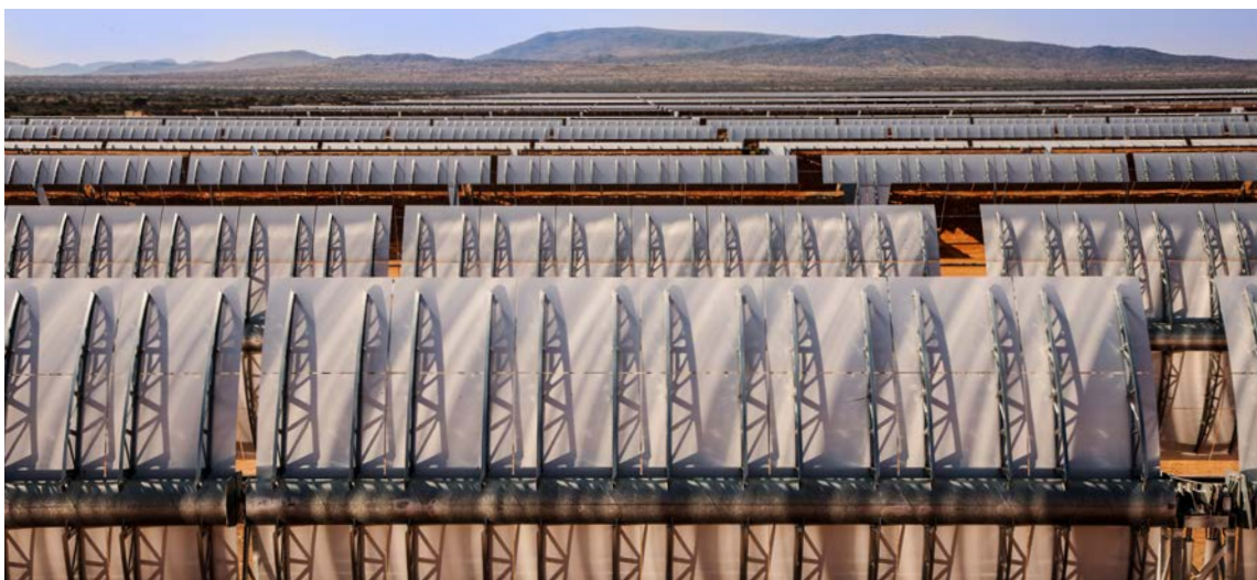
Bokpoort concentrated solar power plant near Groblershoop
