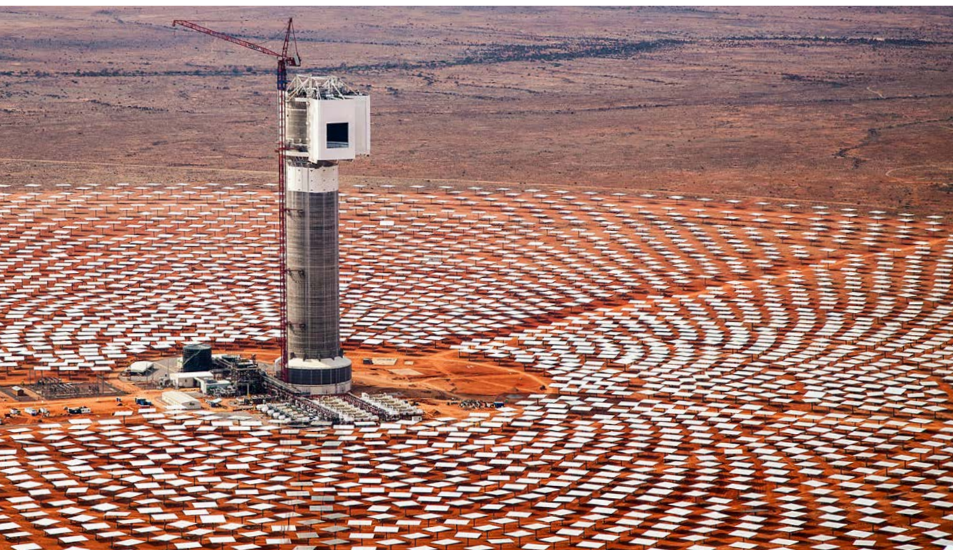
Khi Solar 1 concentrated solar power plant near Upington
