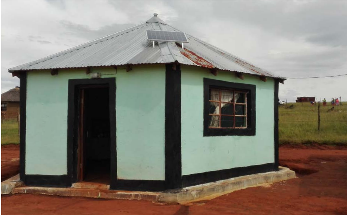
Figure 3: Solar Home System installation, Matatiele, Eastern Cape
