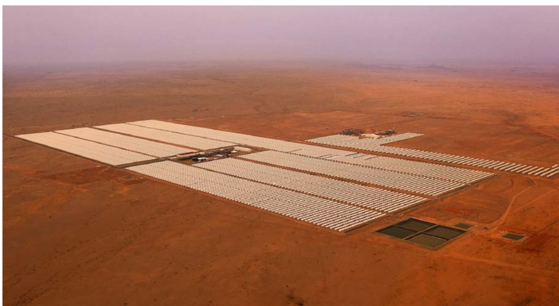
Bokpoort concentrated solar power plant near Groblershoop
