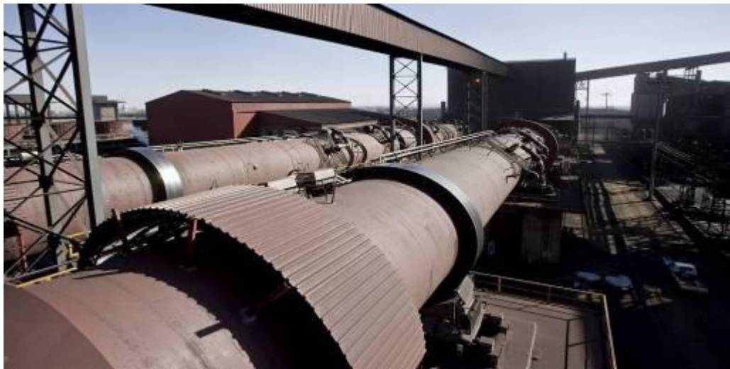
Fig. A.4-4: The general view of the DR Kilns 5 and 6
