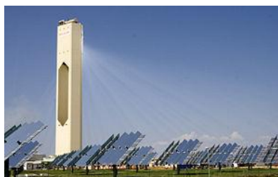
Figure A.4-3: Typical CSP plant (with tower)
