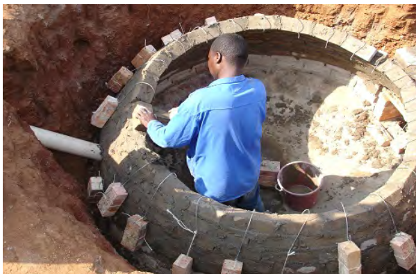
Digester under construction
