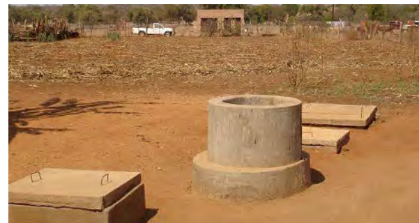
A completed biogas digester
