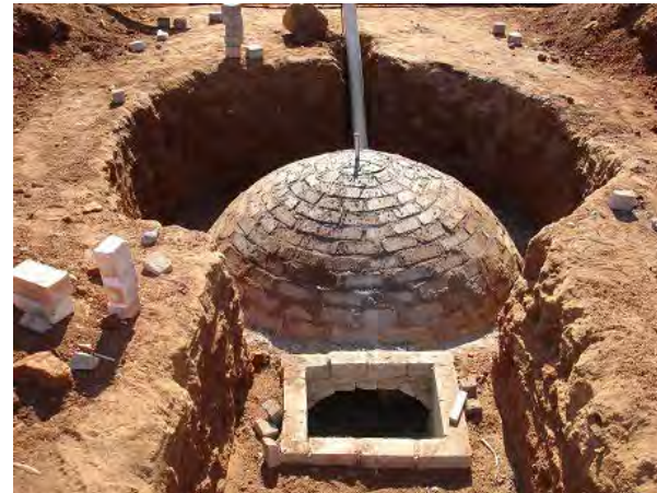
Digester under construction
