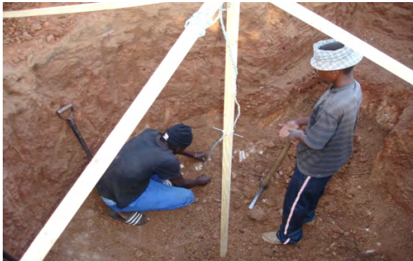
Digging the pit
