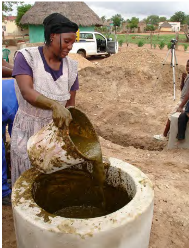
Filling the biogas digester
