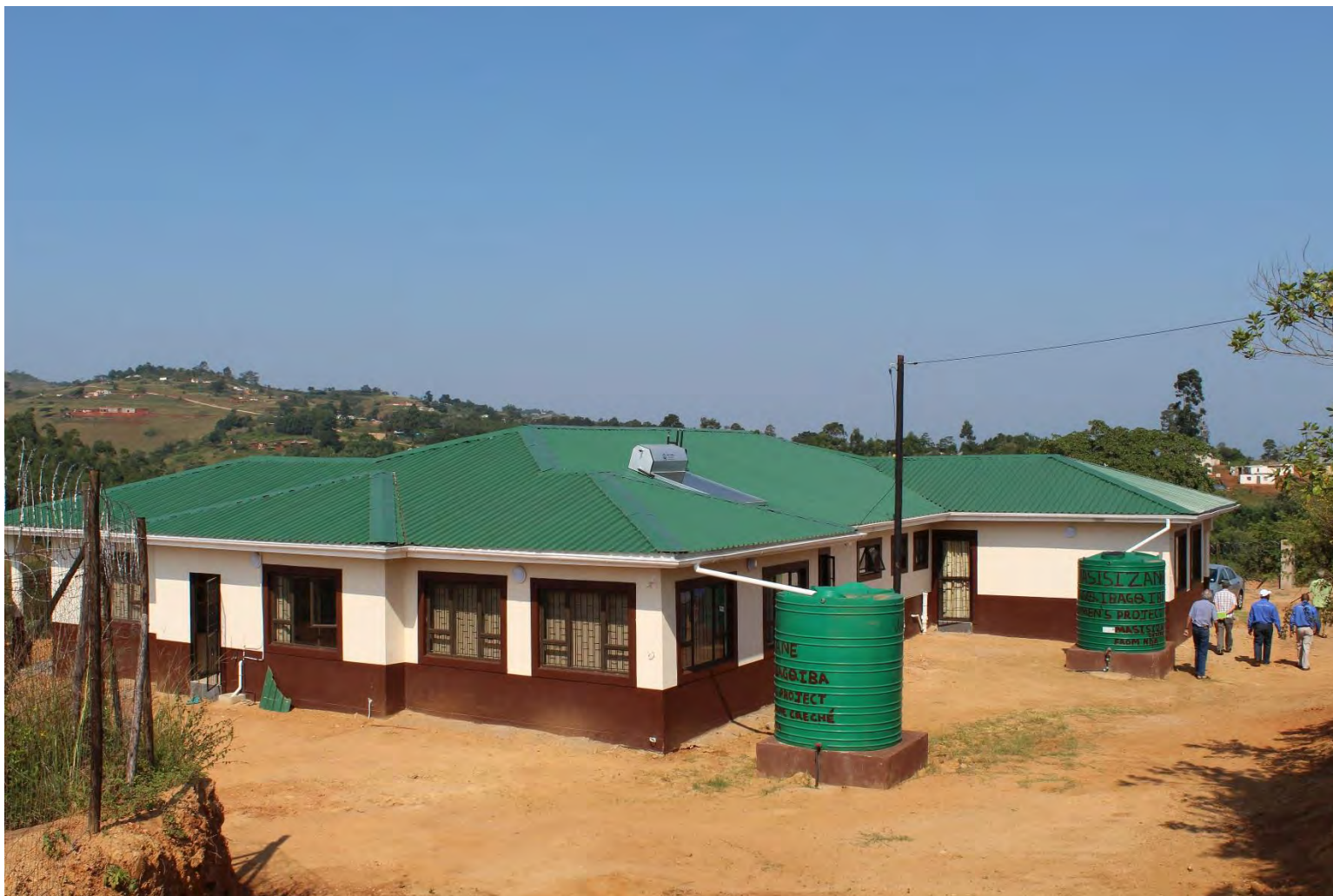
Solar water heating, rain water harvesting, bioenergy, food gardens and efficient lighting
