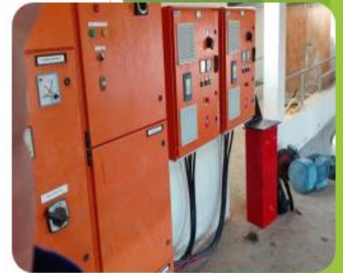
VSDs Installed at Treatment Plant
