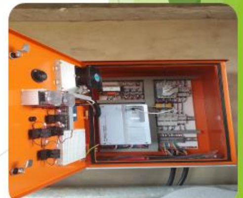
VSDs Installed at Treatment Plant
